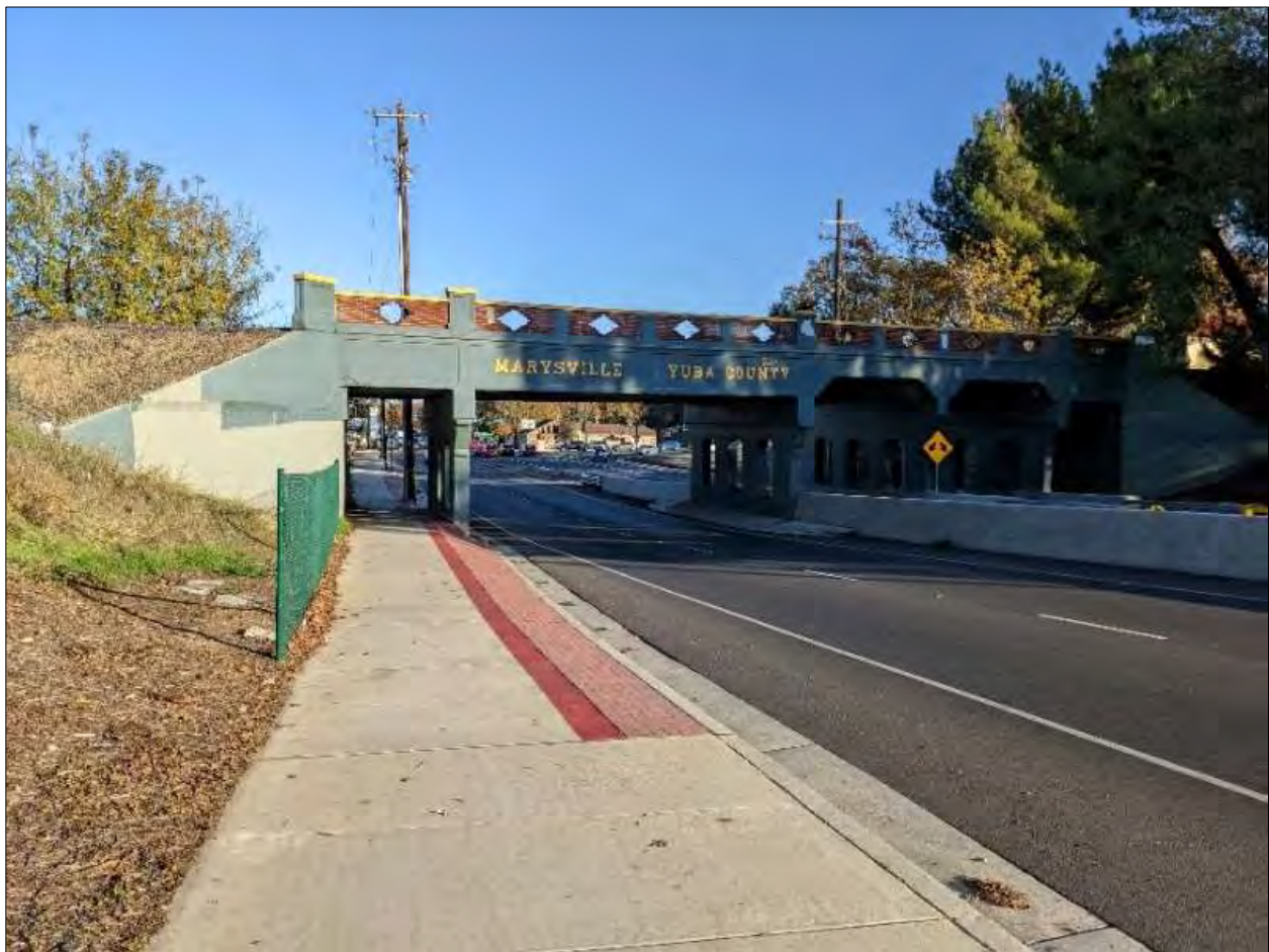
Above: Union Pacific Railroad Overcrossing
