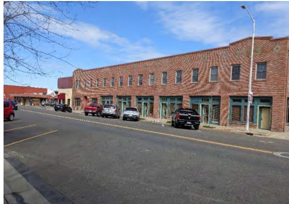
3 rd Street looking northwest toward C Street
